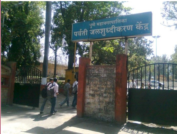
Parwati Water Treatment Plant, pune
